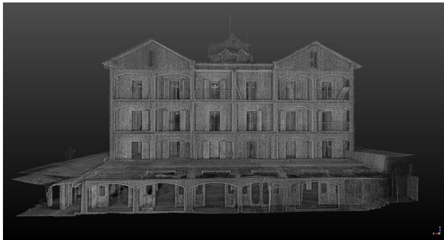
Building surveyed with TIMMS - point cloud by reflectance
